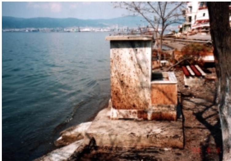
Figure 11.4 Traces of crude oil on the fountain smeared by high sea waves at Hal dere
