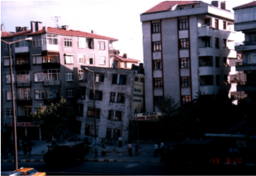
Figure 9.4 Collapsed 5 story RC building in Avcılar (Istanbul)
