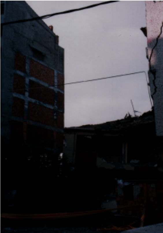
Figure 9.5 Non-damaged reinforced concrete building with solid bricks in T c lar district of Adapazar where liquefaction was widespread
