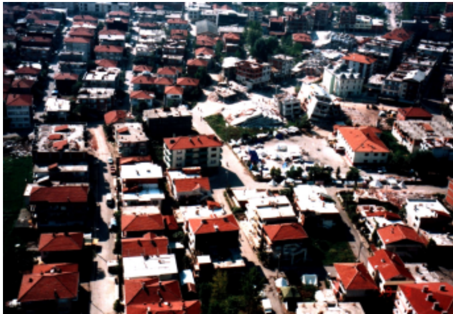
Figure 9.2 An aerial view of collapsed reinforced concrete buildings in Adapazar
