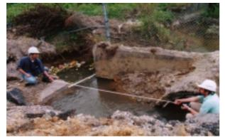
Figure 8.4 Breakage of sewage pipe crossing a main foult
