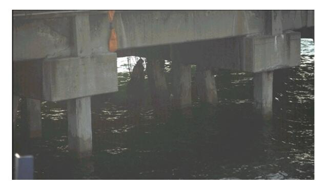
Figure 6.7 RC pile supported dolphine
